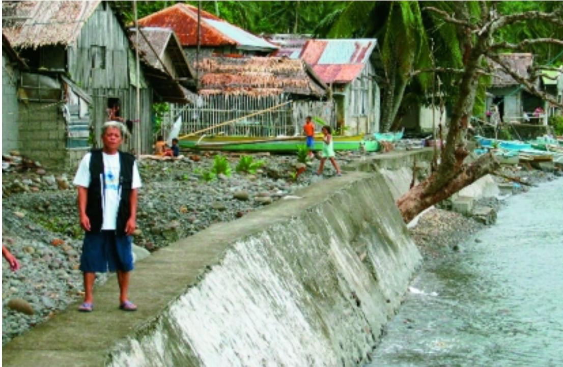
The construction of low seawalls in Son-ok II and Libagon Southern Leyte, prevented damage to fragile houses along the beachfront during typhoons in 2001 and 2003.
