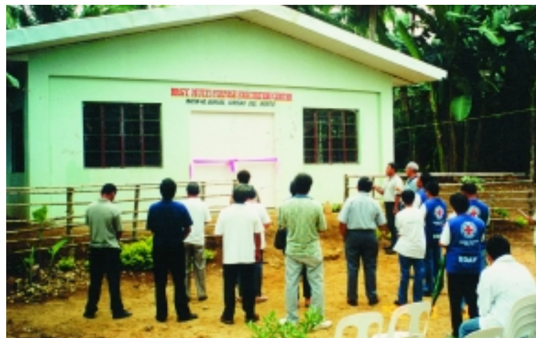
A “multi-purpose evacuation centre” was built in Matin-ao to serve as an alternative school building during annual floods when the old school is not safe. Between floods, it is used for health dissemination and as a clinic when doctors visit the community.
