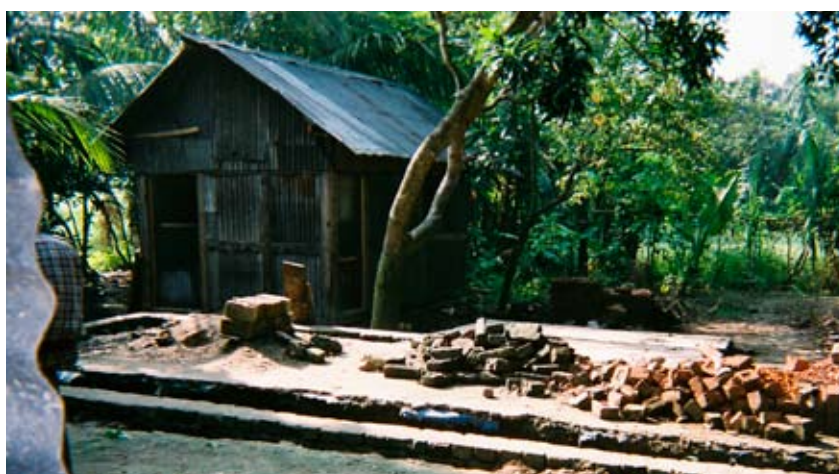
FHH are still re-building their house after Cyclone Sidr (Peri-urban South).
