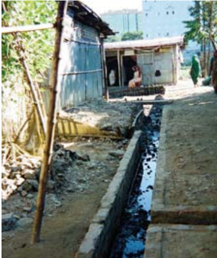
Construction of good drains has improved the disposal of wastewater (North).
